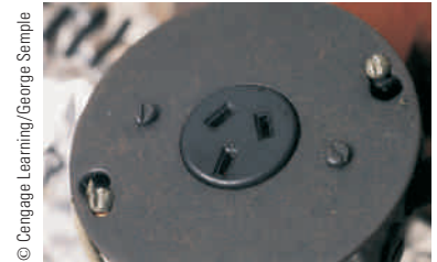
Figure 18.22 (a) The connections for each of the openings in a 240-V outlet. (b) An outlet for connection to a 240-V supply.
